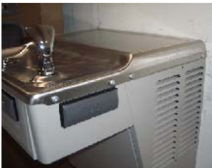
Remove Basin Fasteners
