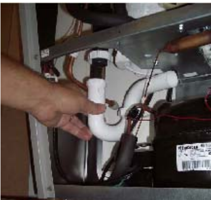
Loosen Drain Line
