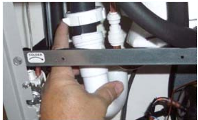
Reattach drain line to P-trap
