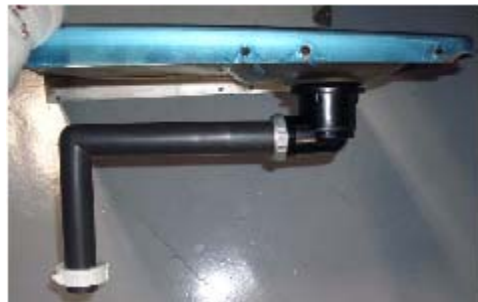
Exchange Drain hardware.
