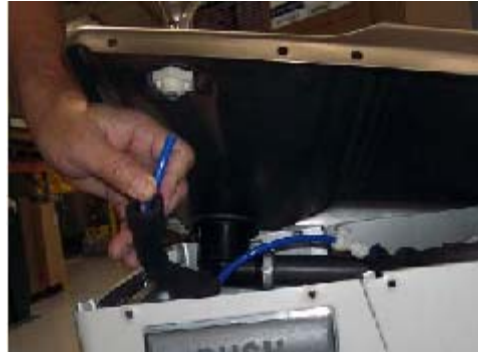
Remove Bubbler Water Line
