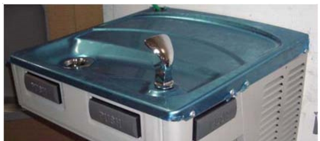
Fasten Basin Assembly in place.
