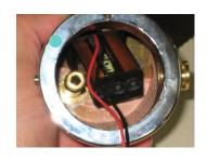
12. Slide the Sensor Assembly with the Capacitor facing into the faucet body cavity and slide the Sensor into the sensor opening. **CARE NOT TO SCRATCH THE LENS.**
