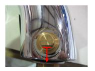
17. Rotate the MV Stem set screw forward in the limiting slot in the forward position and assemble the Set Screw to 1/8 turn tight.
