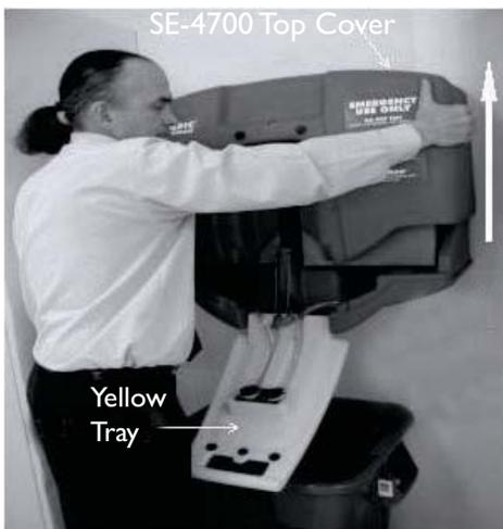
2. Remove and properly discard the old, used cartridges including hoses and spray outlets. The spray outlets are removed from the yellow pull down tray by pressing down the tab in the hole above each outlet and then moving them away from the centerline of the yellow pull down tray.
