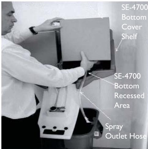
4. Remove and discard the protective bags from the spray outlets. **DO NOT PULL ON CHAIN OR RED CAPS. THIS WILL ACTIVATE THE UNIT AND RENDER IT USELESS.**
